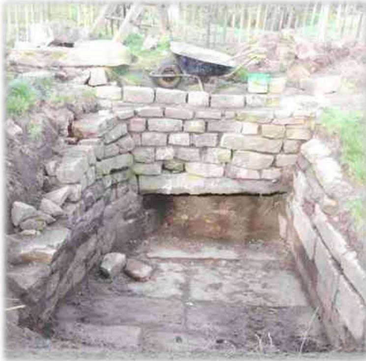
To ensure health and safety we erected chestnut piling given the depth of the mill race. The Parish Lengthsman Tim Hoyles and Pilling's Parish Lengthsman, Graham Armer worked together to reconstruct the walls of the mill race and sluice gate with the stones which had been revealed and a few that had been put away for safe keeping.
